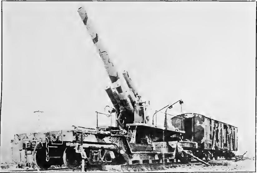
**8-INCH SEACOAST RIFLE, WITH RECOIL MECHANISMS, SET UP ON A SPECIALLY
